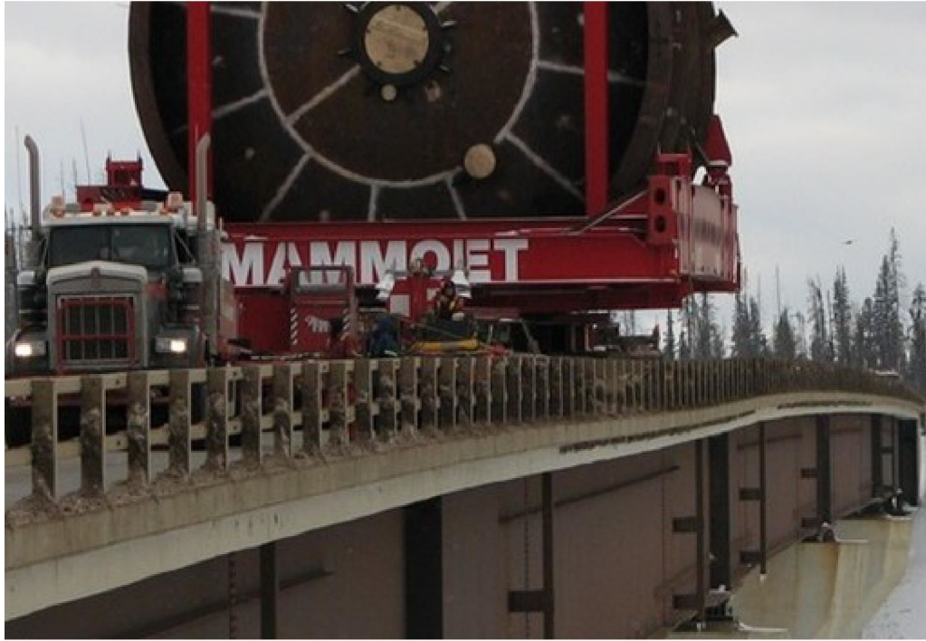
Figure 2-1: Overweight vehicle causing visible deflections in bridge (Lin et al., 2012, p. 23).
